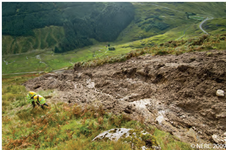
Landslide above A83 at Rest and Be Thankful (Fergus MacTaggart, P710737, British Geological Survey ©NERC)
